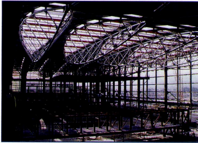
Fig. 1 — The football-shaped trusses at San Francisco International Airport.
